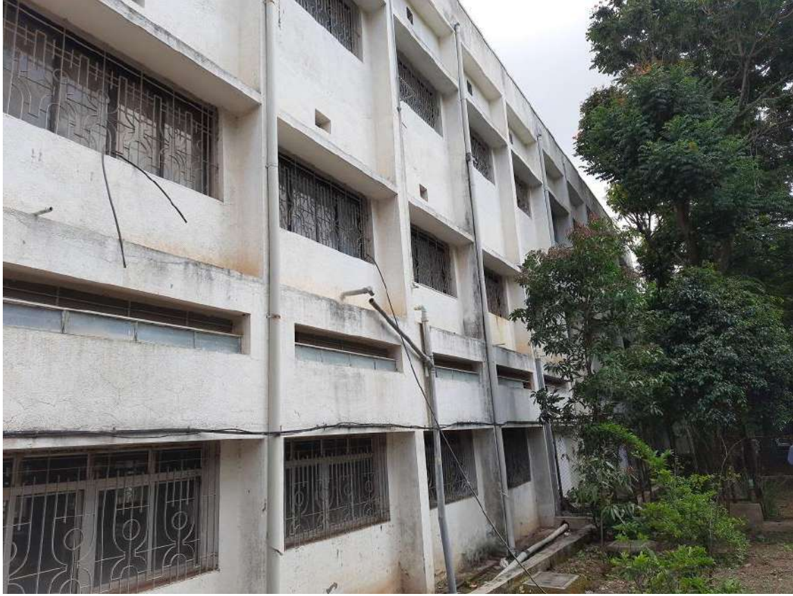
Rainwater harvesting pipelines of college building
