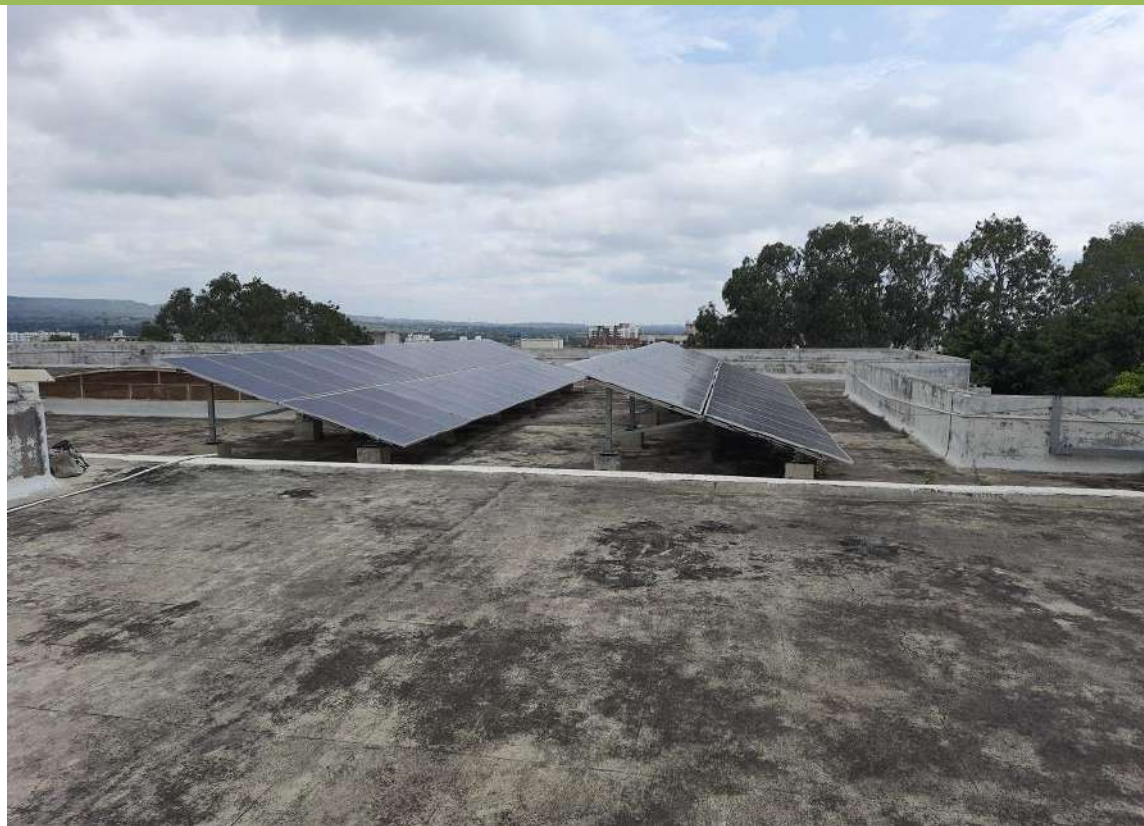
Solar photovoltaic system- 10 kWp College Building
